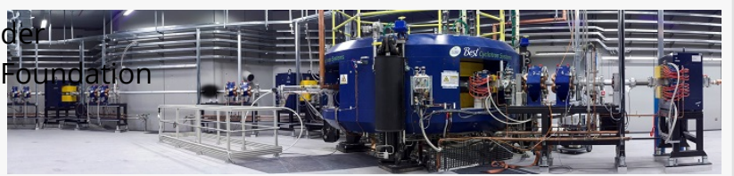
Best 70 MeV Proton Cyclotron installed in INFN, Legnaro, Italy (Photo courtesy of Laboratori Nazionali di Legnaro)
