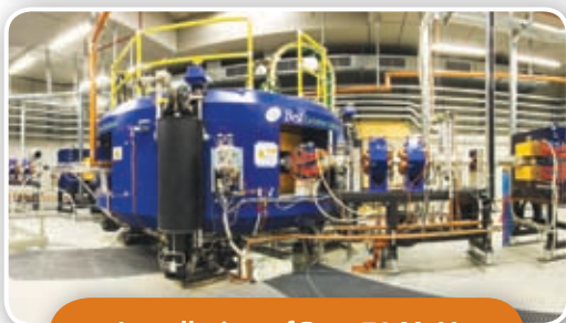
Installation of Best 70 MeV Cyclotron at INFN, Legnaro, Italy
